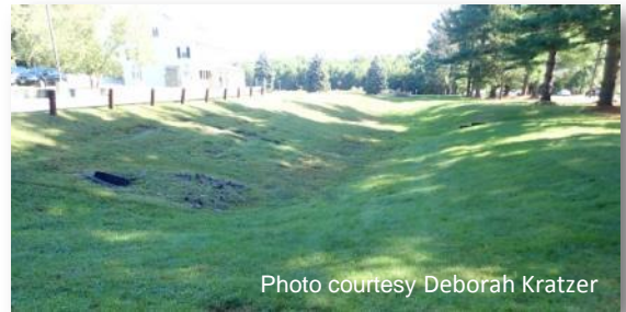
A stormwater infiltration basin by the Ocean Township Library.
